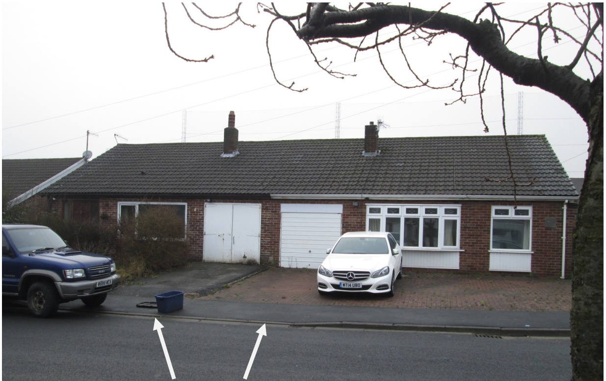
nos. 46 and 48 Lindale Crescent ( as existing)
